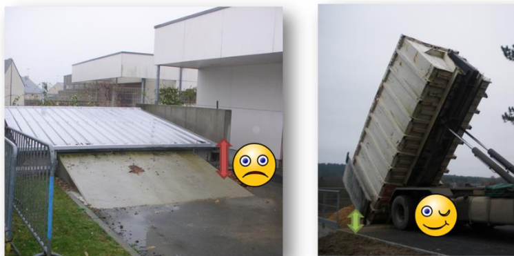
Figure 30 : Example of problematic silo edge configurations - source AILE
