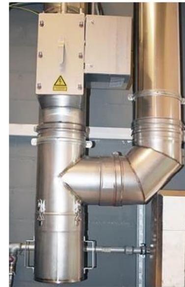
Figure 22: Example of ESP for up to 100 kW [Image source: OekoSolve<sup>21</sup>]
