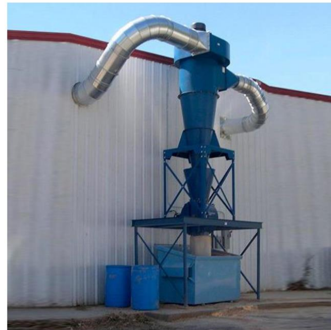
Figure 18: Example of cyclone [Image source: Indiamart.com ]
