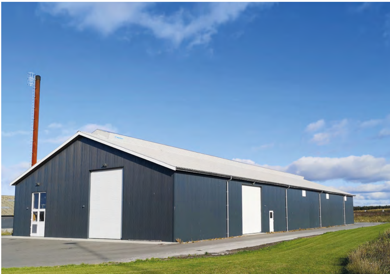
Since the 1980's there has been a decentralisation of Danish energy production, and today many smaller plants generate electricity and district heating. PHOTO Kirsten Krogh.
