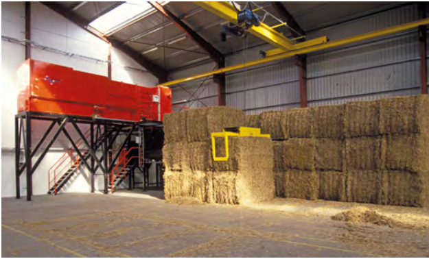
Straw stockroom at Terndrup district heating plant. The transport from the stockroom to the boiler takes place with an automatically controlled crane. The stockroom can contain straw for about one week's operation during winter. PHOTO Torben Skøtt, BioPress.
