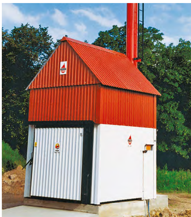
Portion plants are often installed in a separate building in order to reduce fire risks. PHOTO Torben Skøtt, BioPress.
